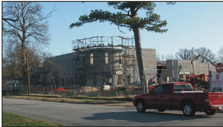
Bentonville Public Library under construction.
