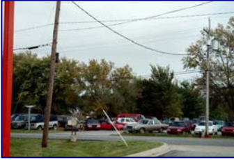
Overhead utility lines
