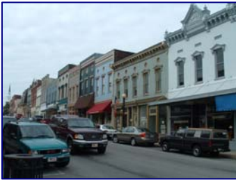
Small town in Kentucky where overhead utility lines have been placed underground
