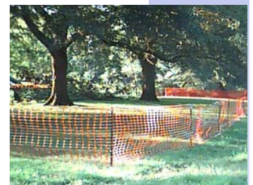
Protective measures such as fencing to prevent compaction of the ground over roots can help trees survive construction. (Policy PE-22)
