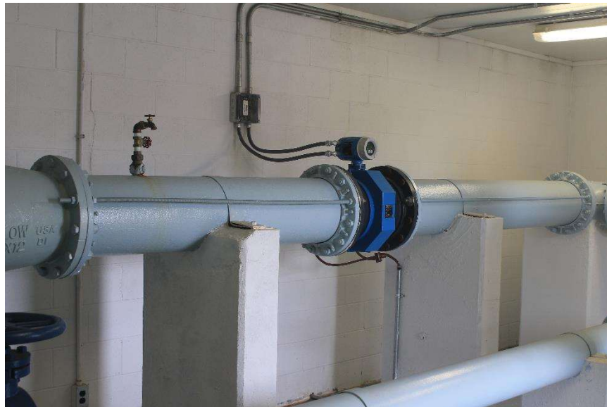
Figure 2-4: Moberly Lane Emergency Connection Meter
