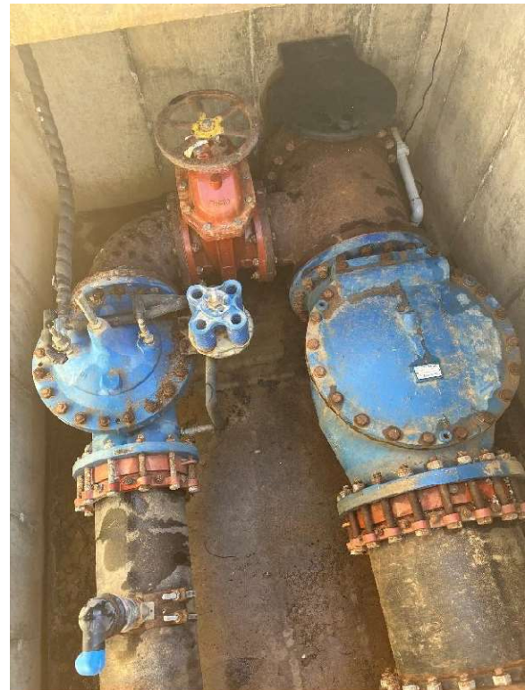
Figure 2-6: Highway 102 Altitude Valve
