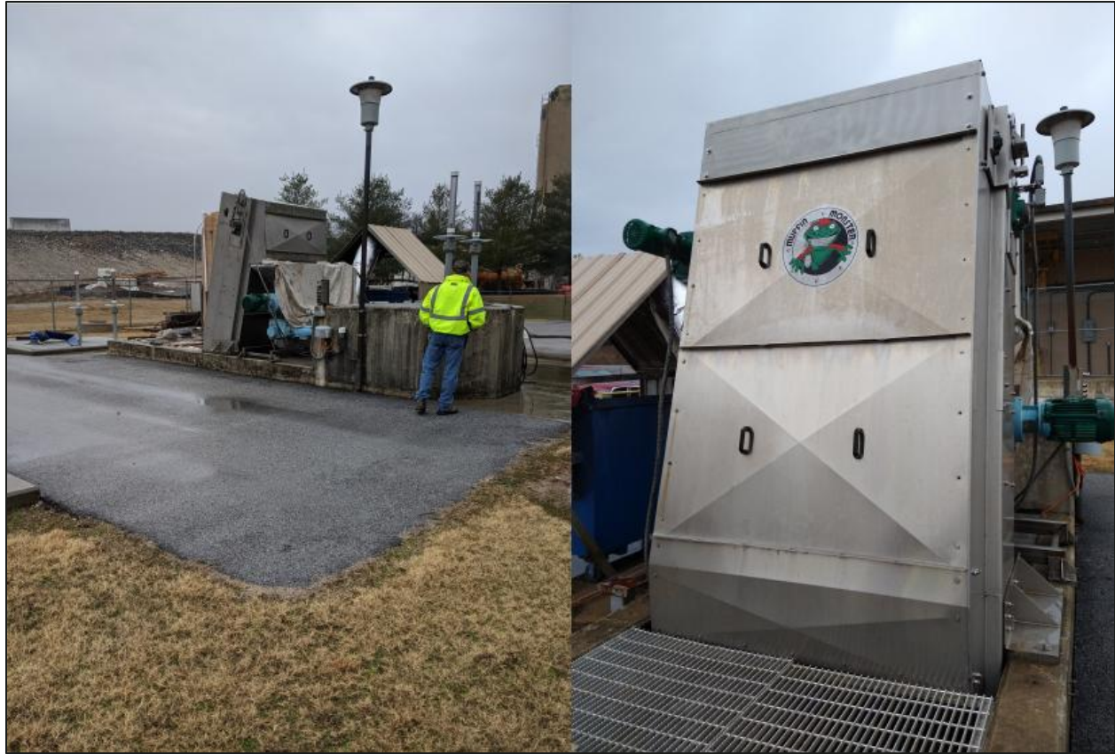
Figure 2. Dogwood Diversion Box and Bar Screen
